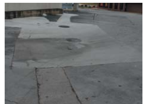
TYPICAL ISOLATION SLAB CONSTRUCTION OVER A GREASE INTERCEPTOR AT A COMMERCIAL SITE.
